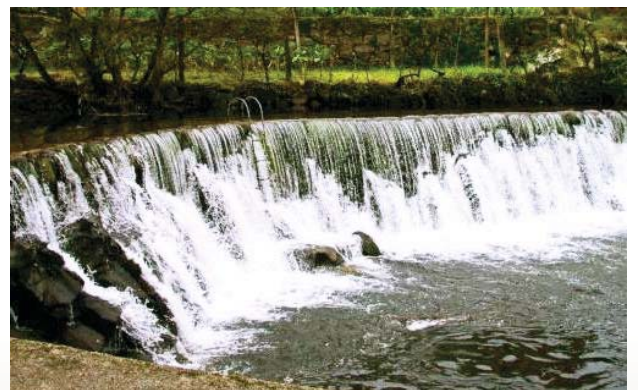
A view of the weir at Cativelos on the river Torto
